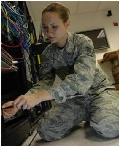
Senior Airman Holly Durkin, a Cyber Surety Technician for the 129th Communications Flight, Moffett Federal Airfield, Calif., replaces an uninterruptable power supply (UPS) from a network server, August 4, 2010. The UPS serves as back-up power supply for network servers in case of main power loss. (Air National Guard photo by Tech. Sgt. Ray Aquino)
